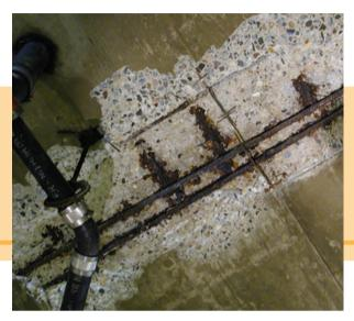
Road salt has caused corrosion of structural rebar and columns throughout the garage.
