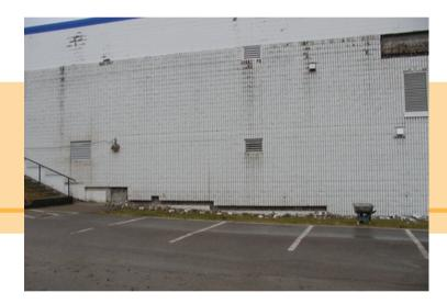
Exterior block has been repaired but continues to fail due to age and lack of a vapor barrier.
