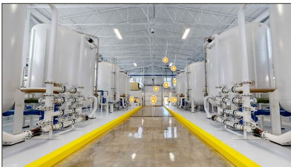
GAC treatment vessels to remove PFAS
