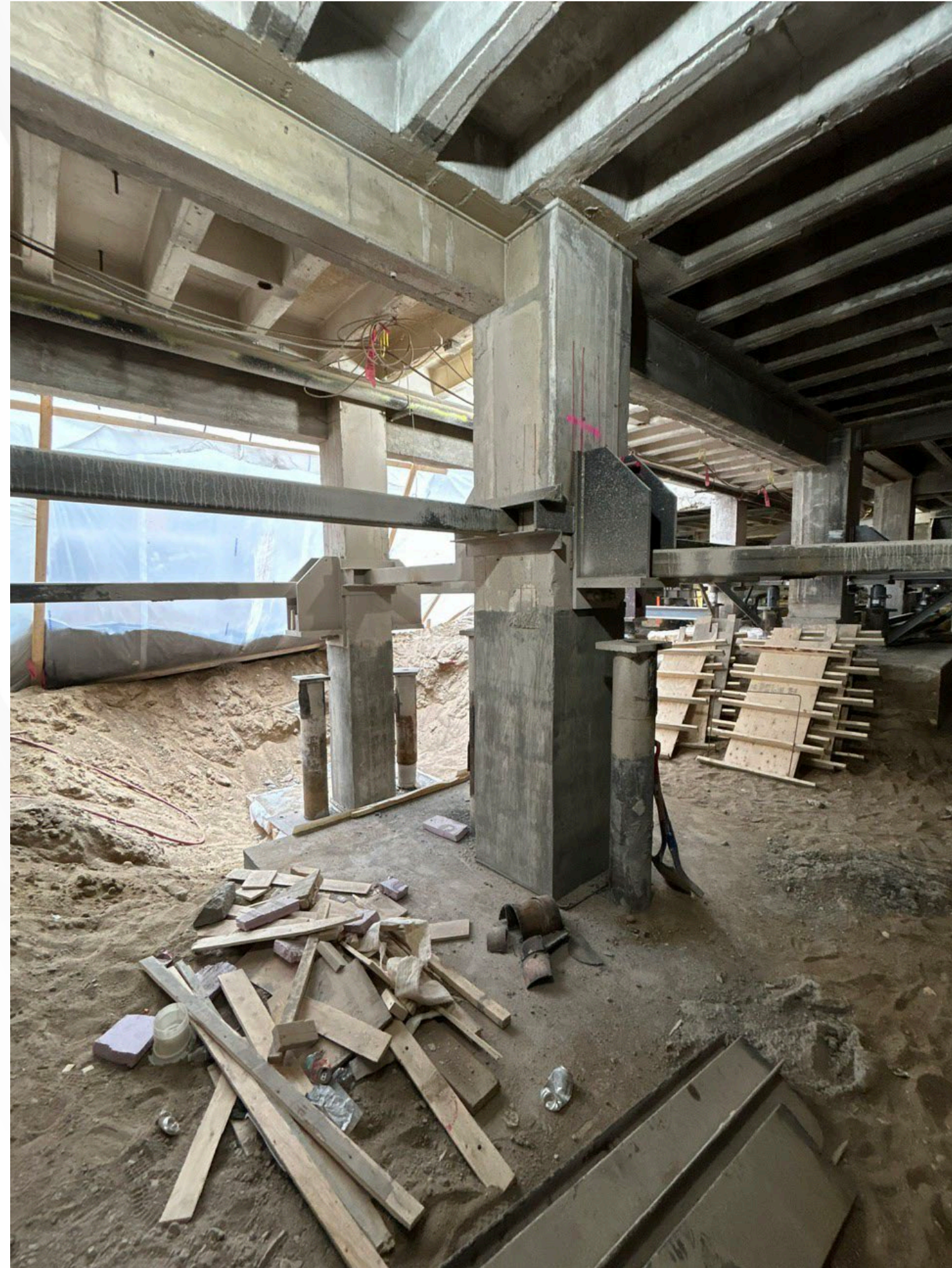
View of column lowering in the Basement Z3
