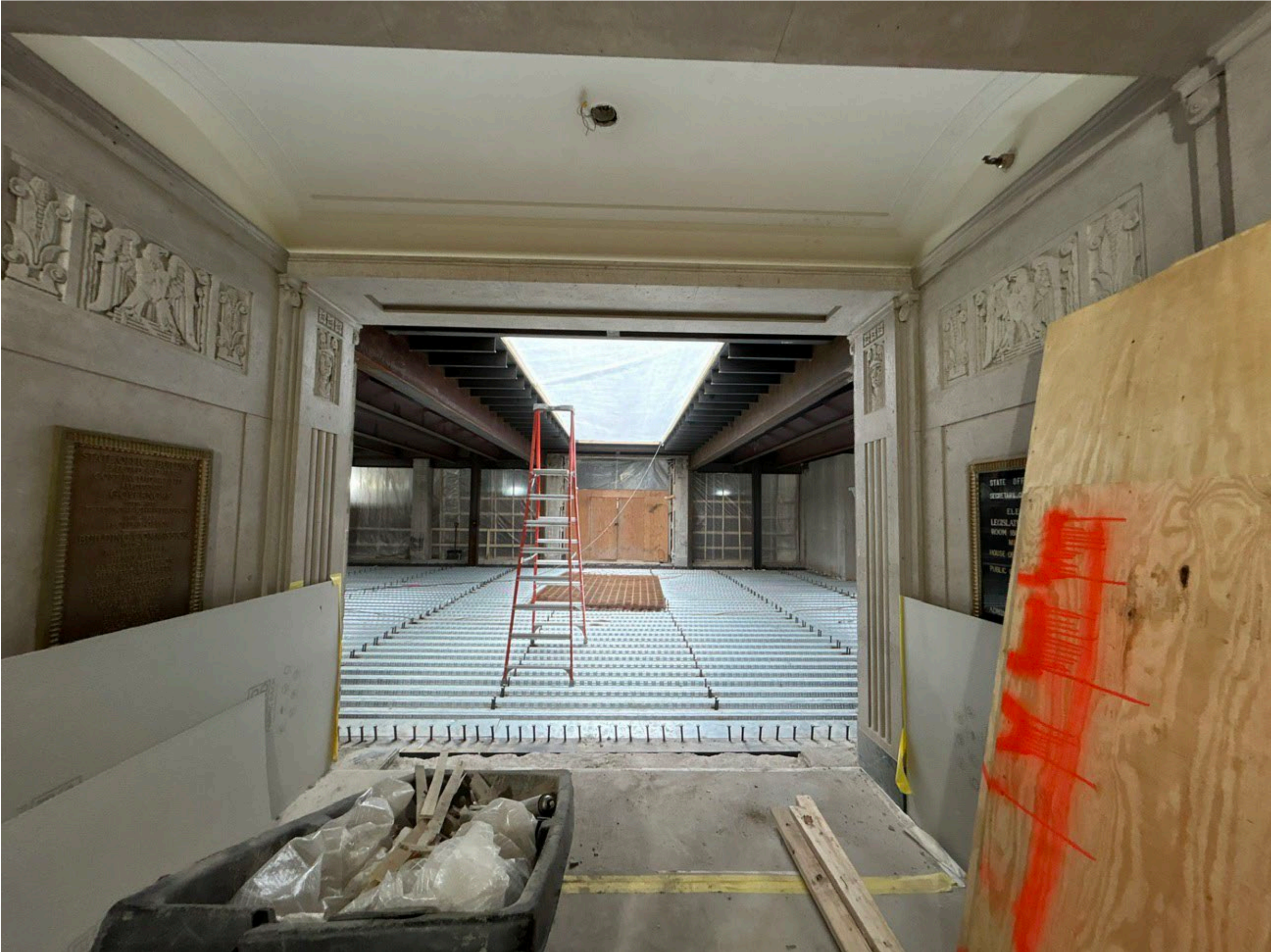
View of 1 st level metal deck and skylight of east courtyard
