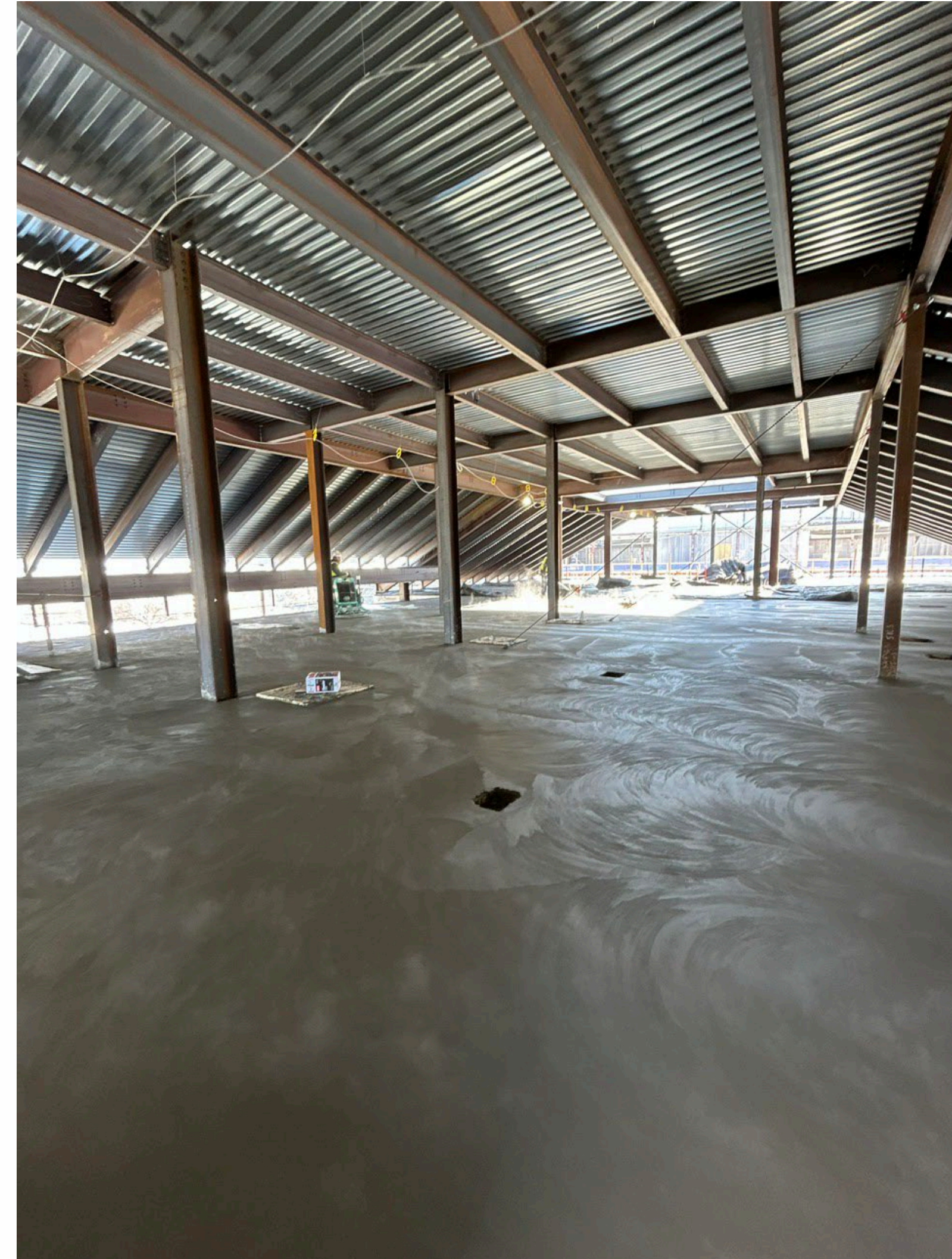
View of Concrete slab on deck at 6 th level of Zone 2
