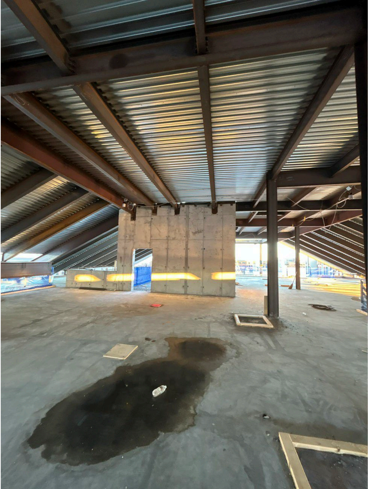
View of 6 th floor cast in place wall
