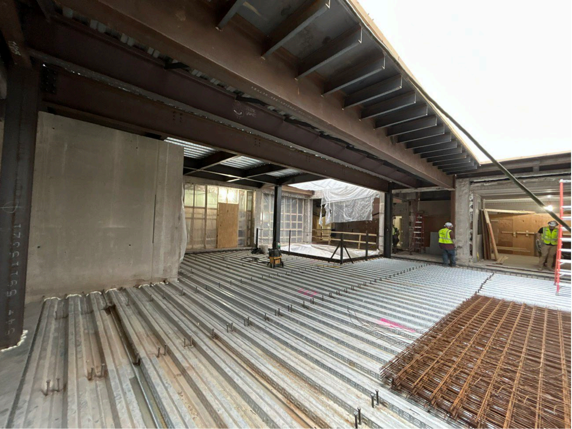
View of 1 st level framing of east courtyard
