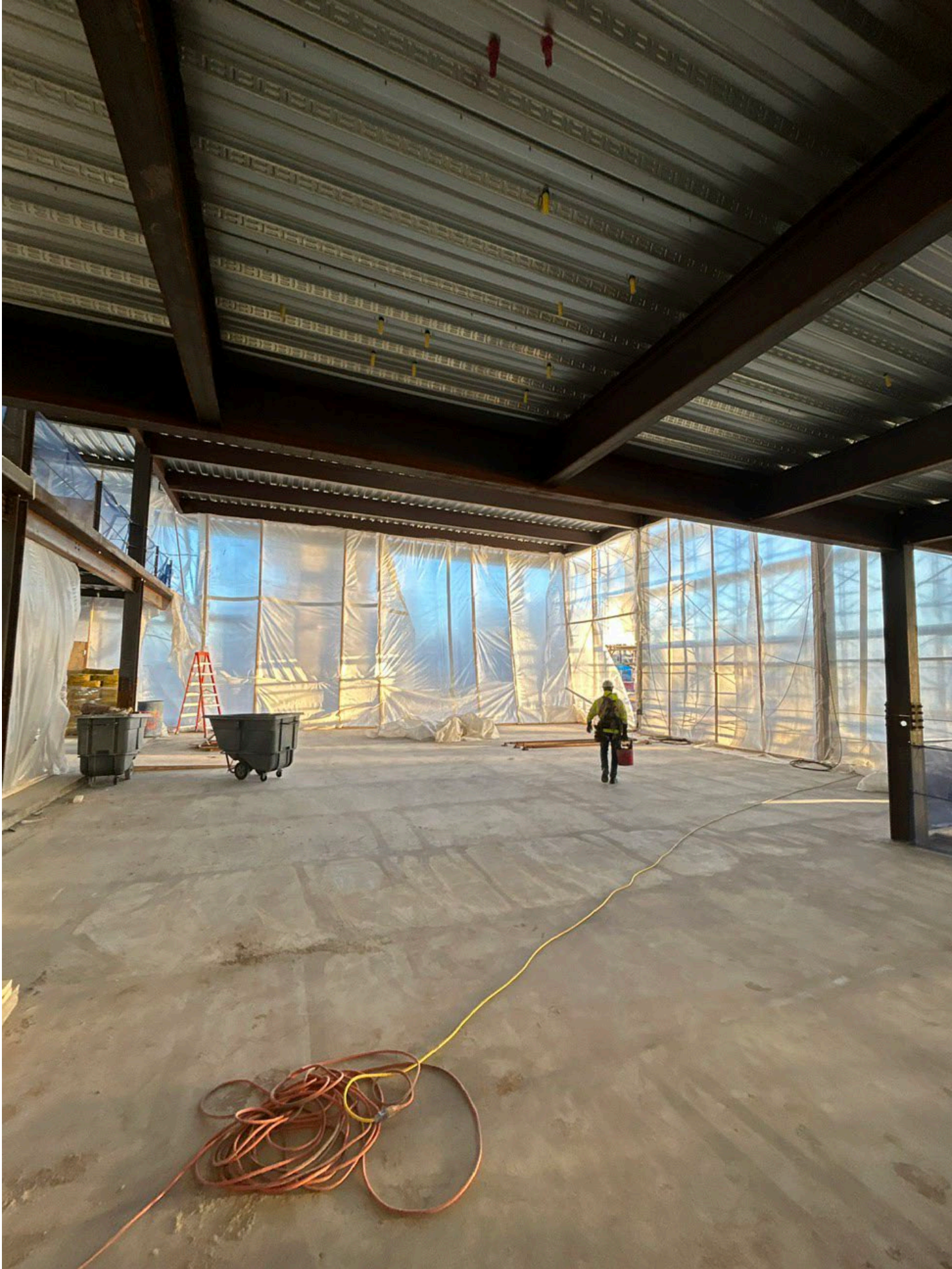
View of medium hearing room 3 rd level looking north
