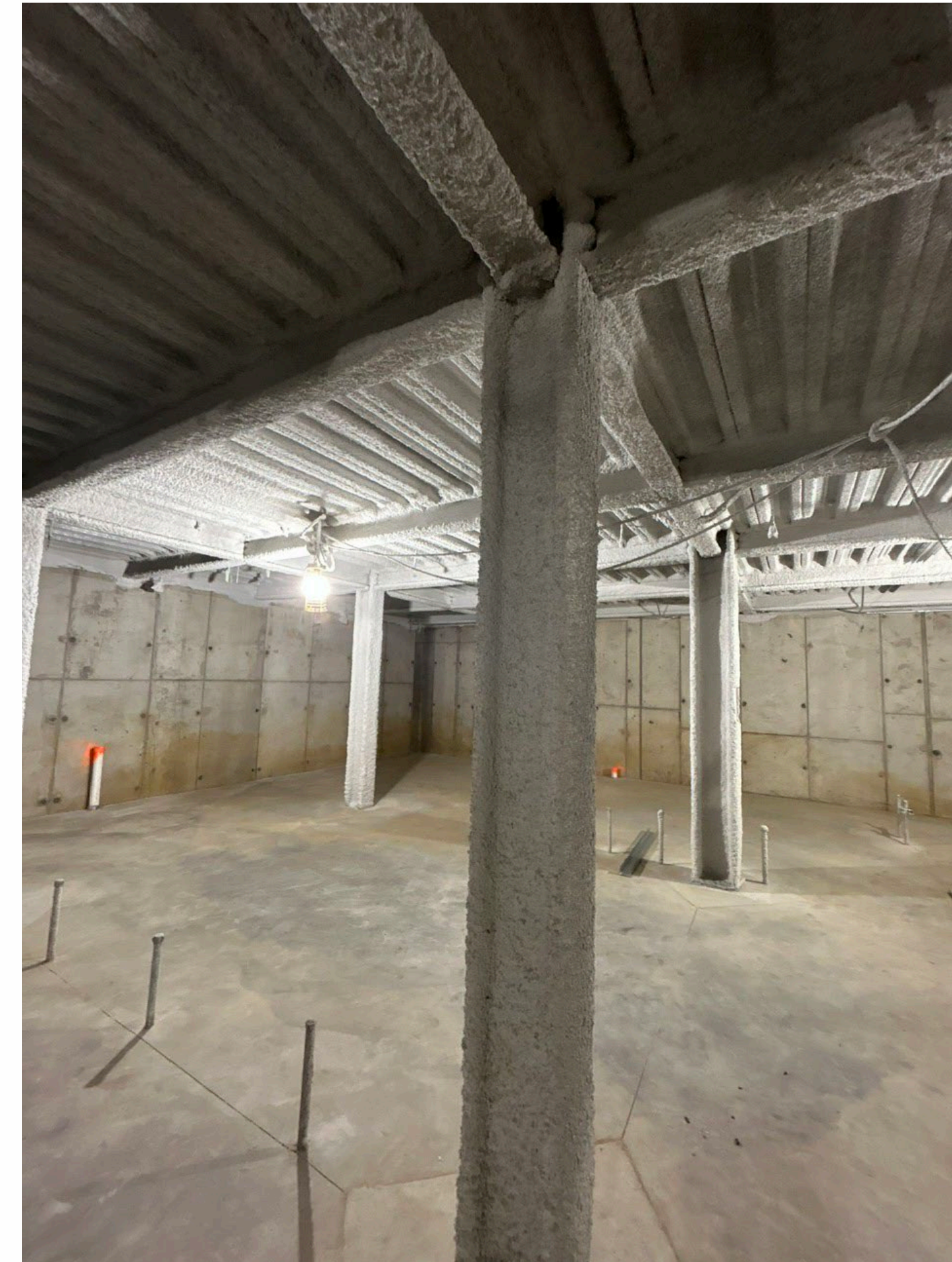
View of fireproofing of beams and columns in Zone 2 Basement
