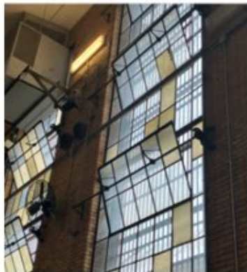
"Temporary" window replacements in yellow
